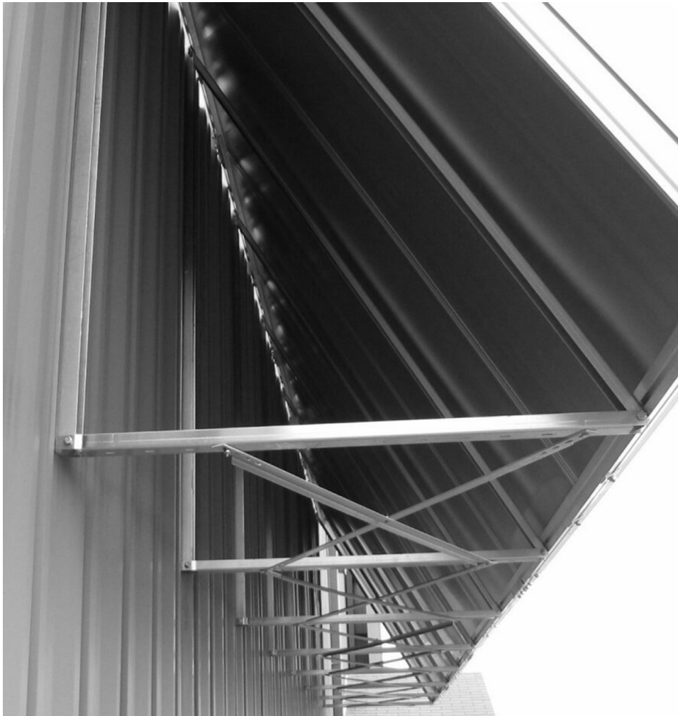
Figure 5.4.5: Typical wall-mount installation of a 60° collector array.
